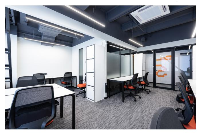
The cassette air conditioners in the office. The main advantage of the cassette split systems is the uniform distribution of air flow in four directions, which allows using only one air conditioner to evenly cool a large room.
